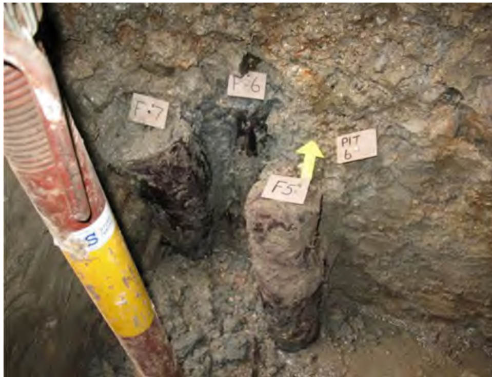
Figure 3 Three wooden piles beneath church tower.
