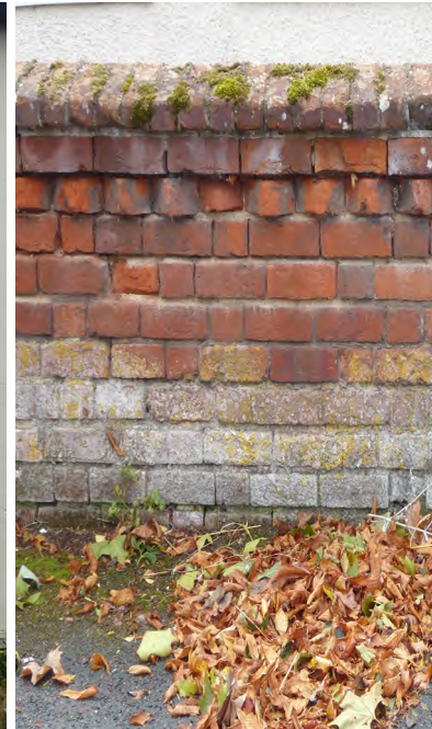
Figure 33 Traditional low brick wall surrounding the church hall
