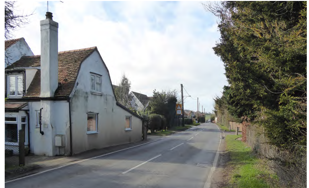
Figure 11 looking west showing Number 45 The Street
