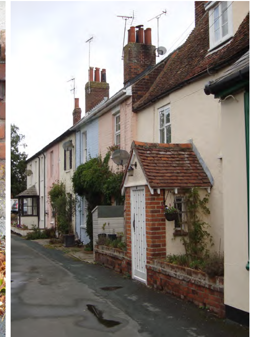
Figure 34 Terraced housing behind the green including Post Office House
