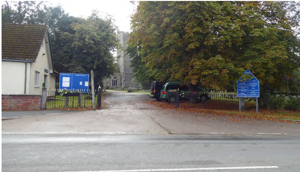
Figure 45 Photograph of the church and approach from The Street
