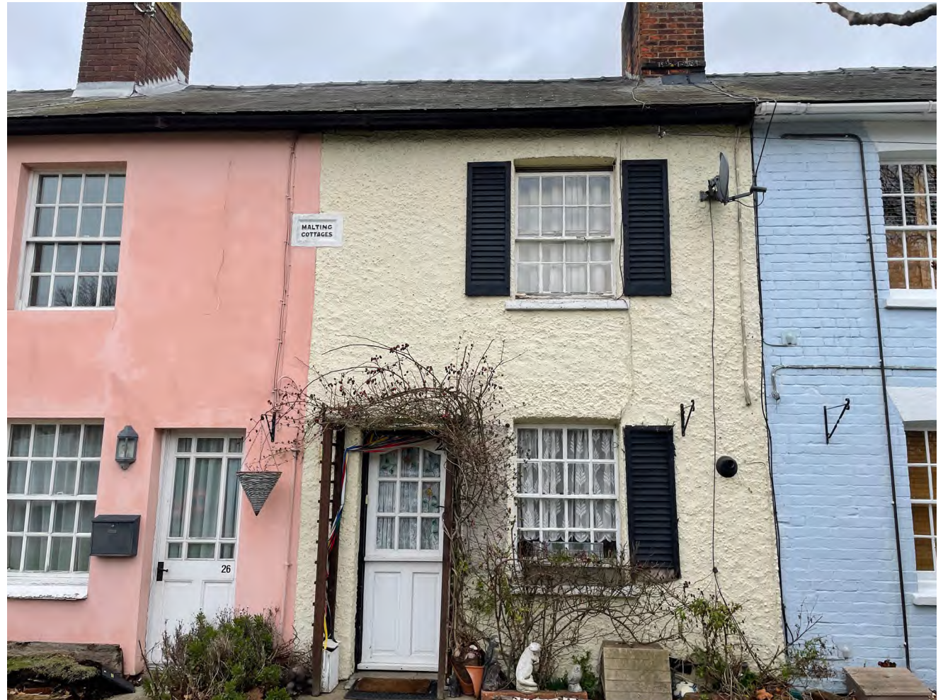
Figure 21 Close up of maltings Cottages
